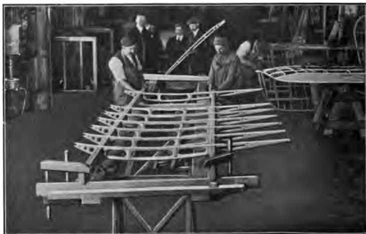
FIG. 131.—Assembling wing with spars.
